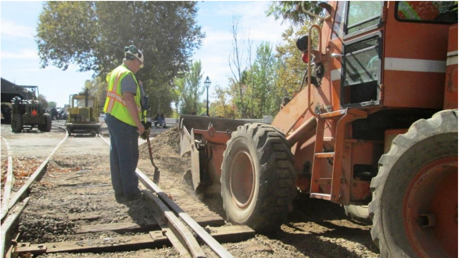
Chris gives Al in the loader some guidance in trying to cut away as much dirt from around the ties as possible
