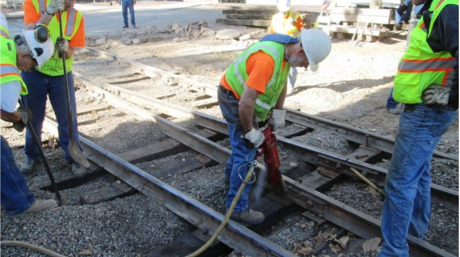
Mike M. driving a spike with the pneumatic spike-driver
