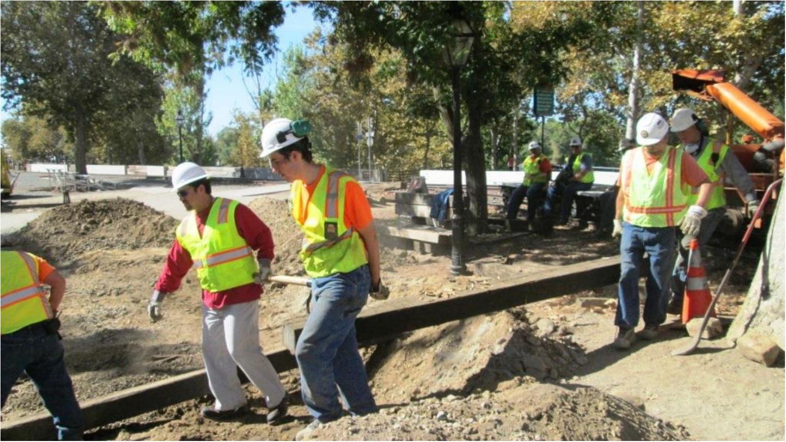
Round 2 and Jose, Weston, John, and Steve bring in a heavy 14-foot long hardwood tie
