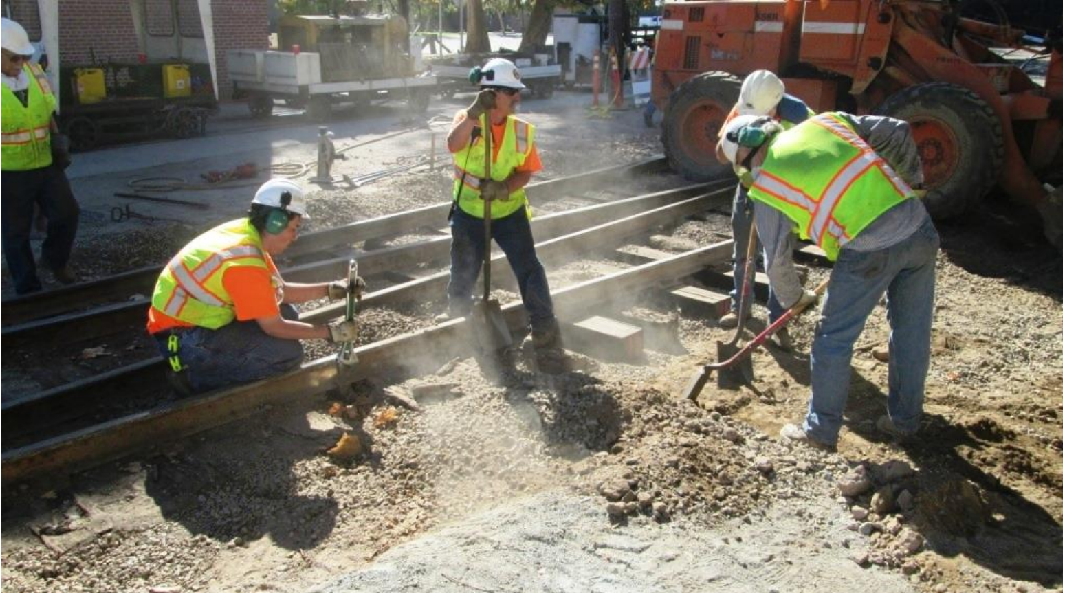
Weston removes a gauge-rod as Joe, Steve, and Mike M. back-fill around the newly inserted tie
