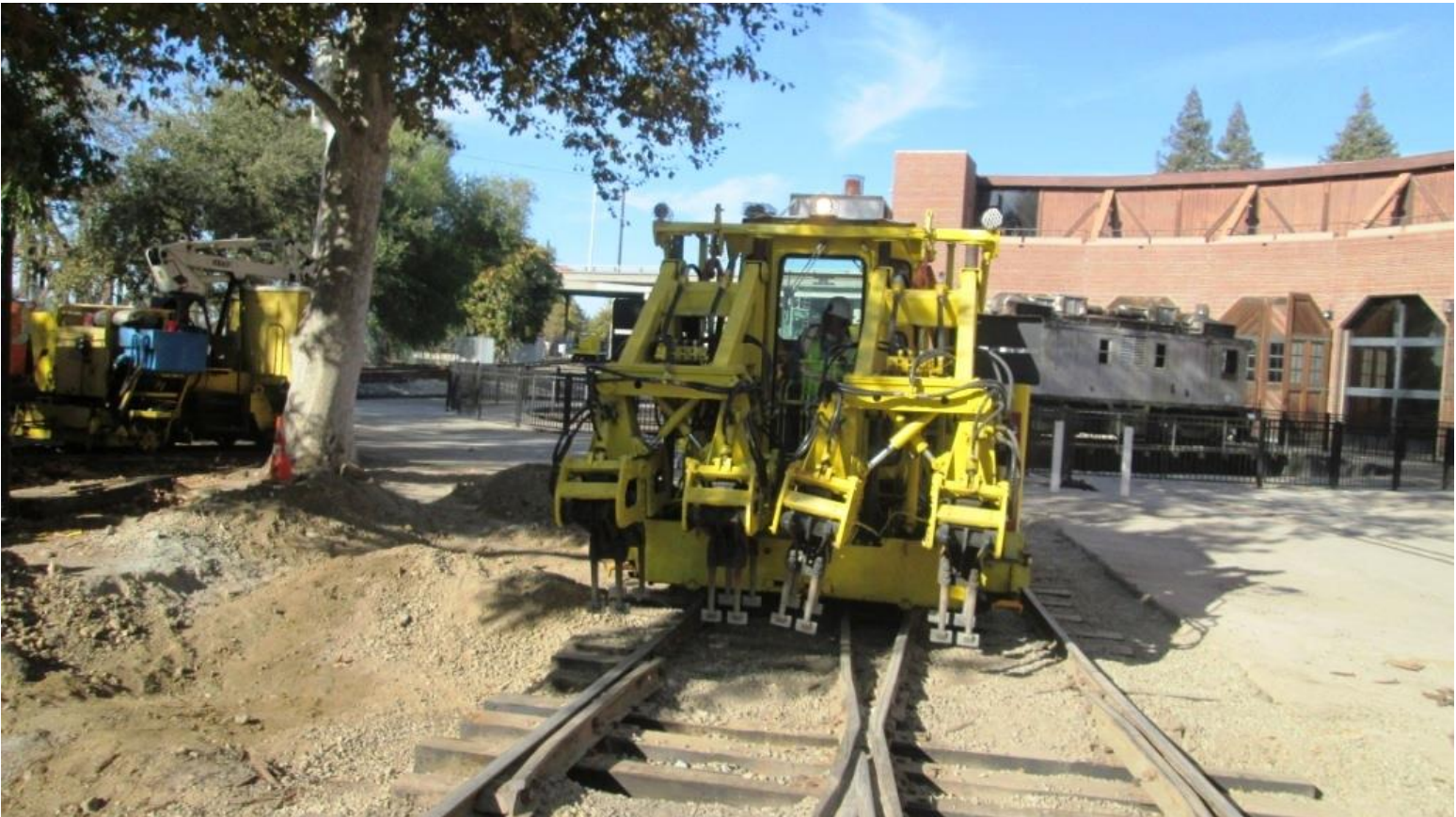
Steve in the tamper expertly maneuvers the work-heads around the converging rails
