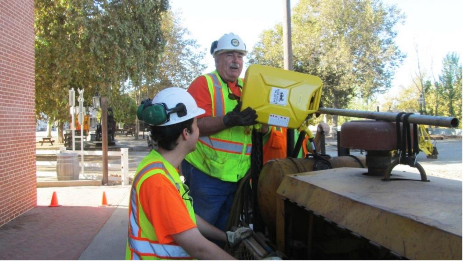
Jedi Master Harry instructs Padawan Weston in the finer arts of adding diesel to the compressor
