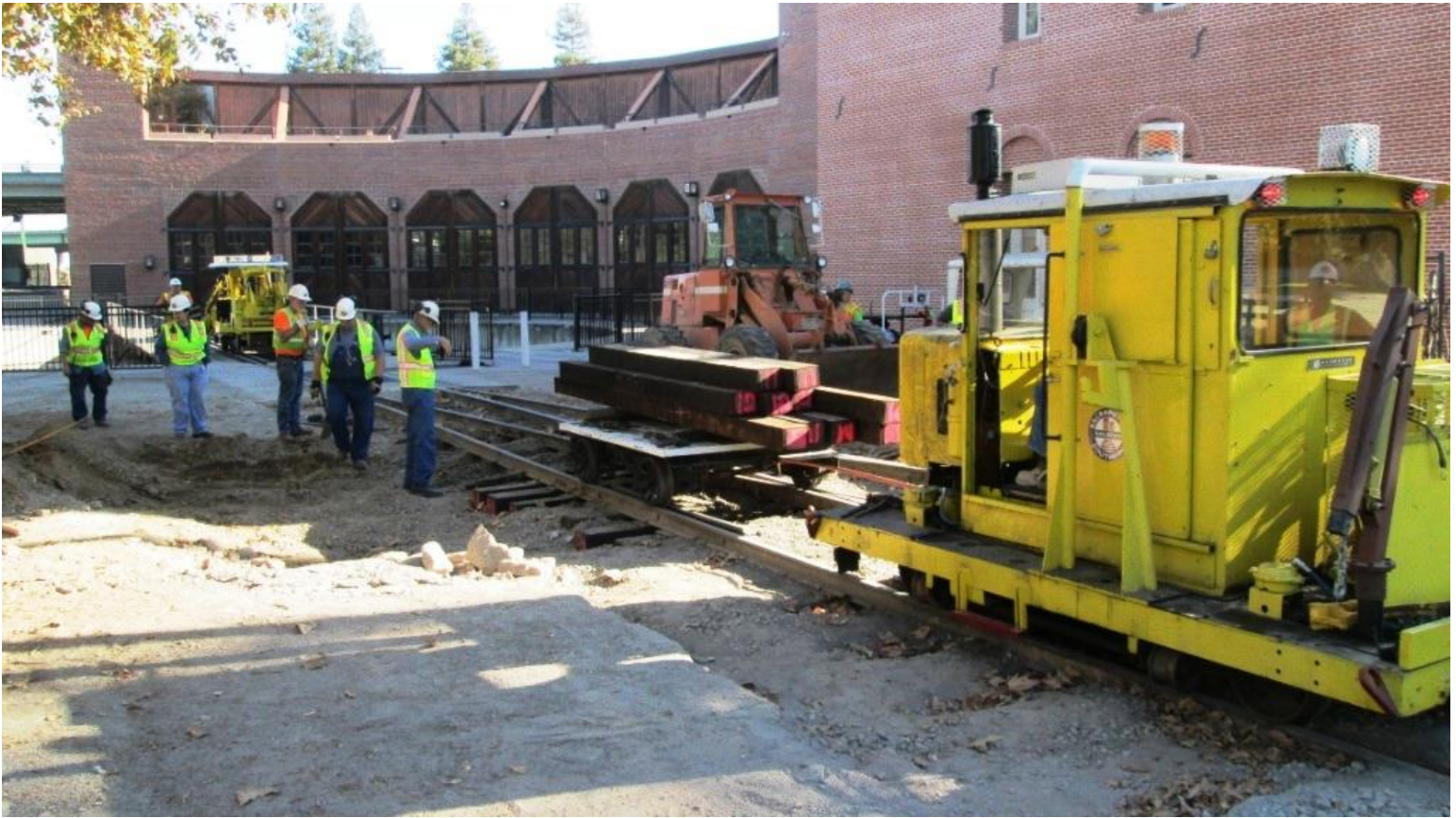
Alan guides Ed in the Kalamazoo shoving the switch-tie laden fiat car
