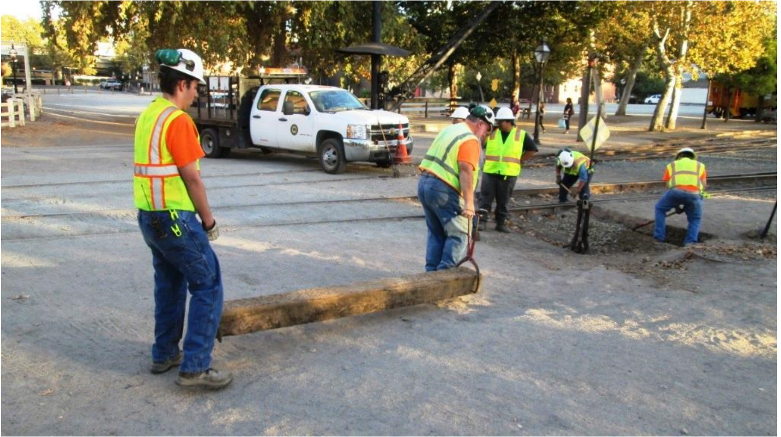
Weston and Frank bring the retaining tie over to the pit around Switch 2
