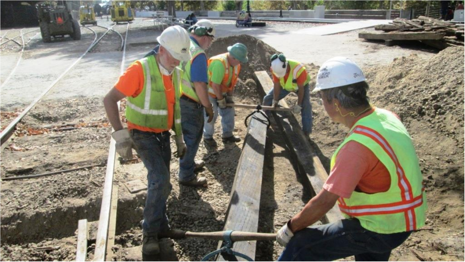
Mike M., John, Frank, Al, and Ed make the Herculean effort to move this massive timber
