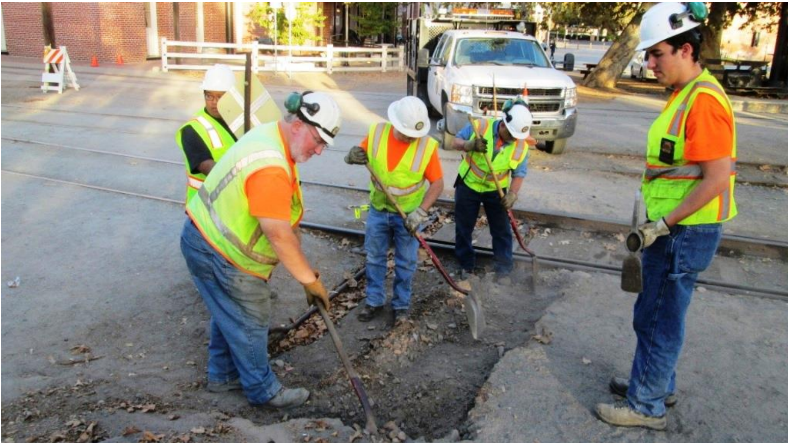
Frank, Mike H., Joe, and Weston clearing out the fallen dirt around the Switch 2 switch-stand
