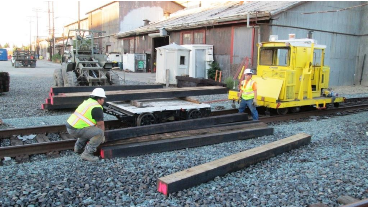
Anthony and Joe positon 14-foot ties onto the flat-car
