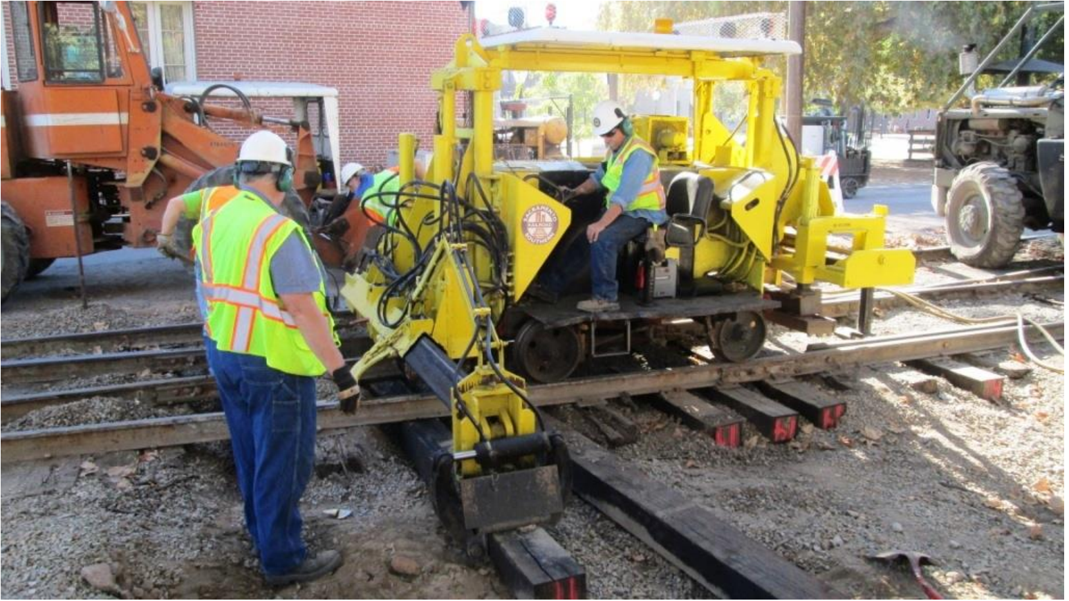
Chris provides Joe on the 125 with a little guidance from the ground as he pulls switch ties under the rails
