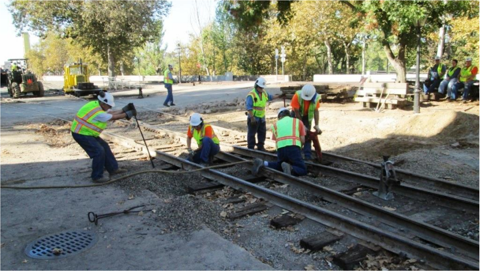
Clem nips the east rail as Weston sets spikes. John sets spike on the west side while Mike M. gets ready to drive them into the ties
