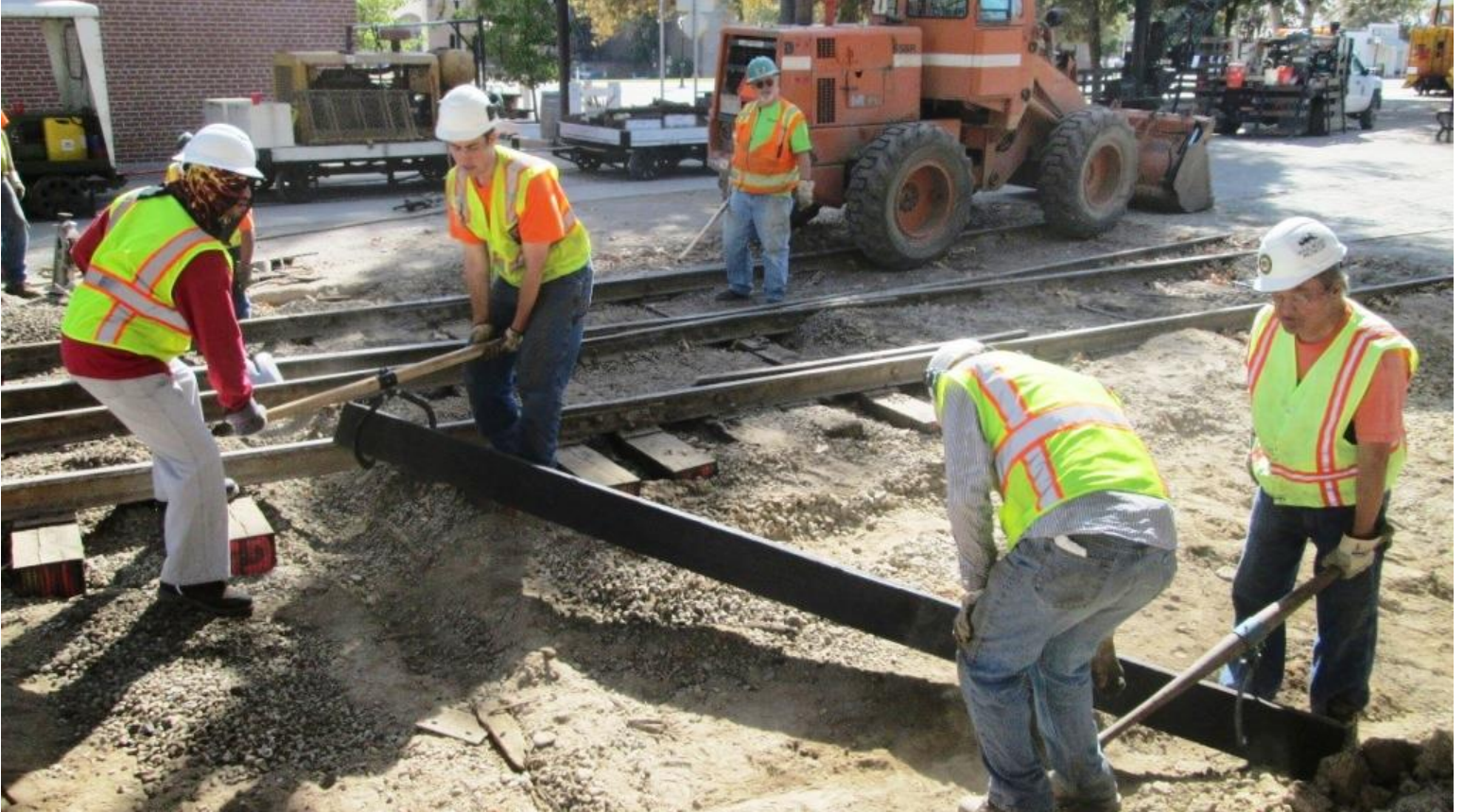
Then, they get it lined up for insertion under the rails
