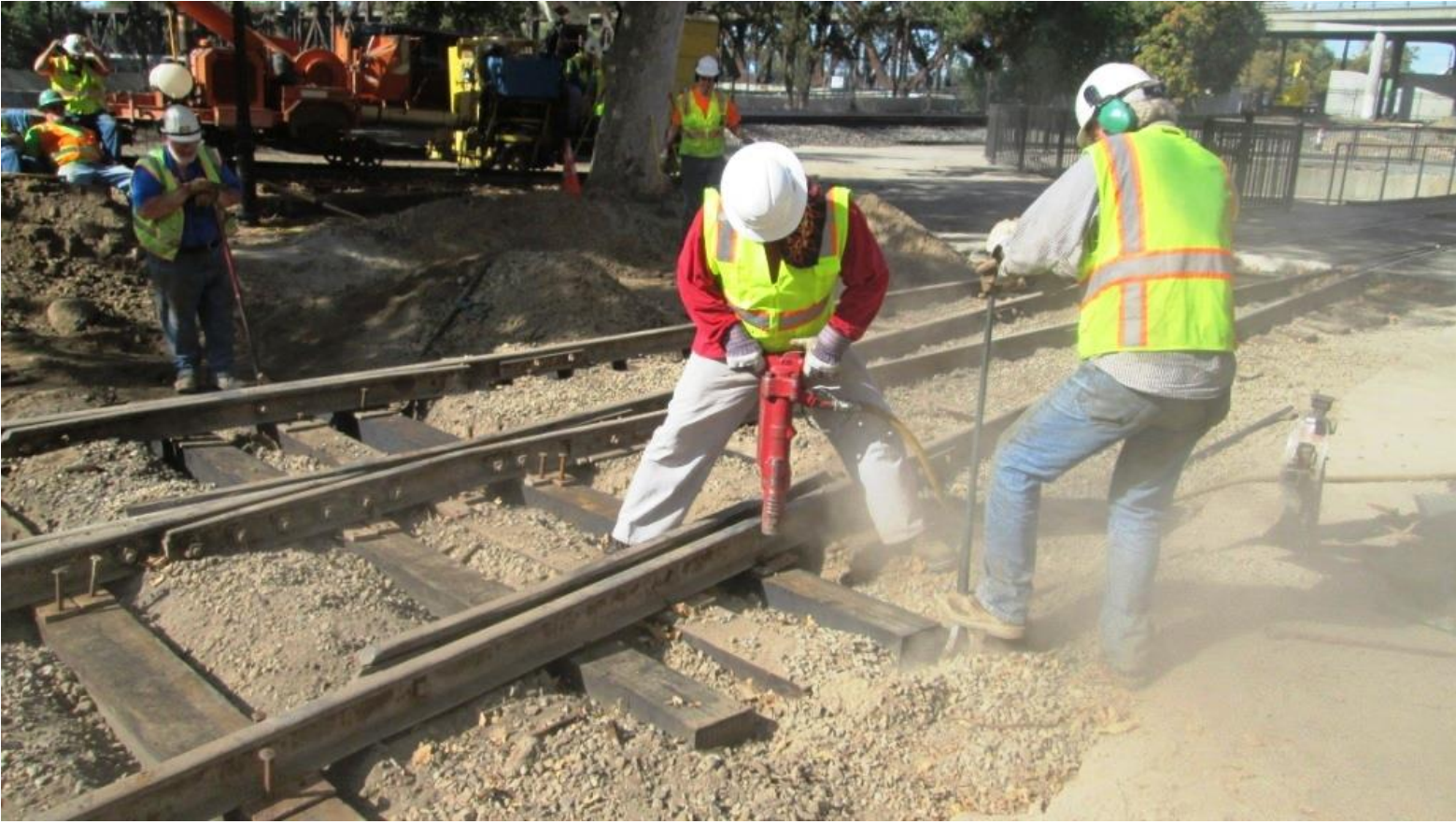
Steve nips the tie as Jose drives a spike
