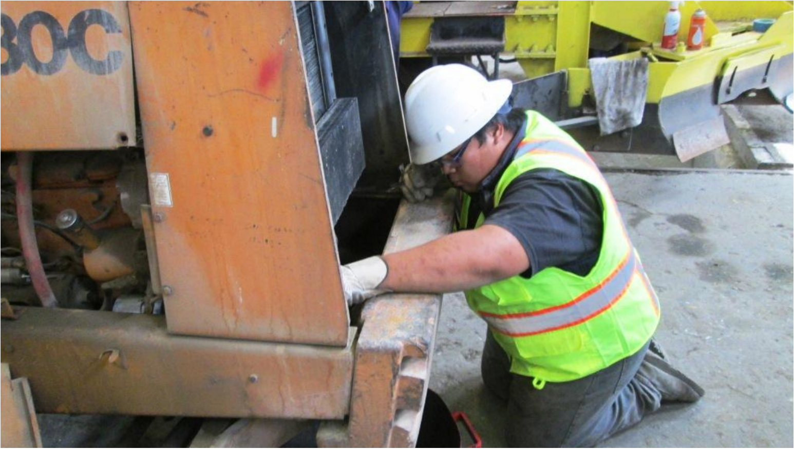
Anthony works to disconnect the shroud over the engine compartment of the back-hoe
