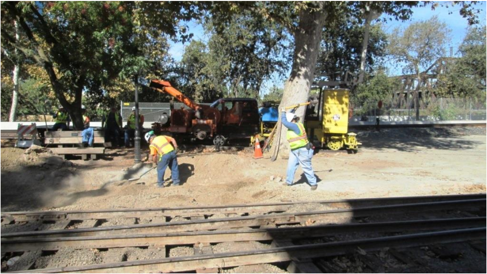
Heather takes out her frustrations by beating the soil-cement into submission
