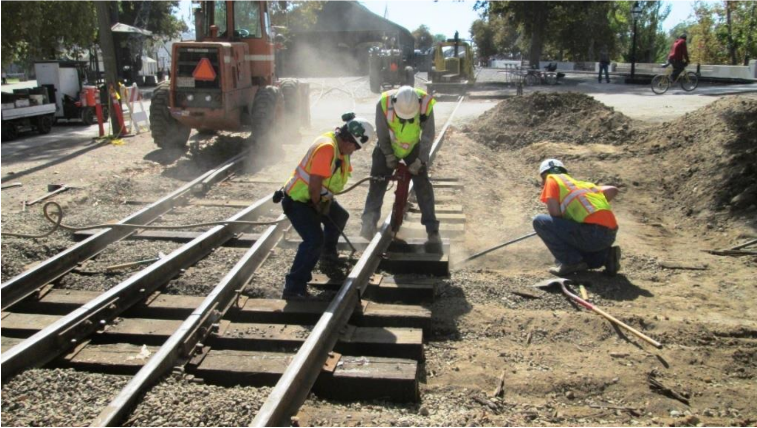
Joe and Weston nip-up the tie as Steve drives the spikes
