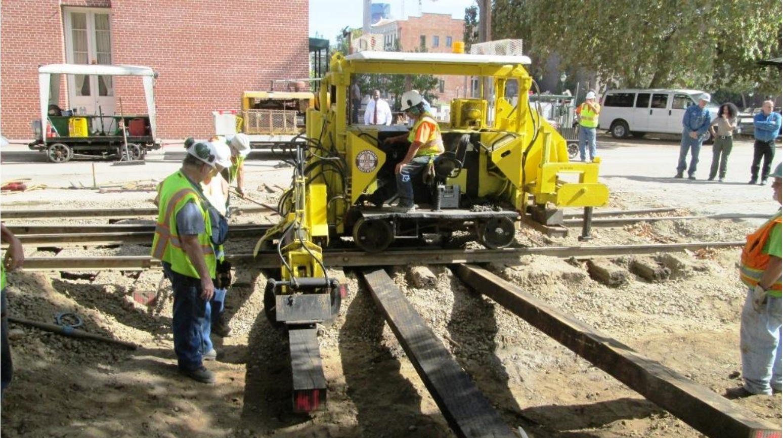
Joe pulls another three ties under the rails
