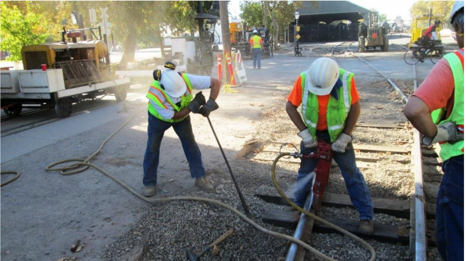
Clem nips-up the tie as Mike M. drives the spike
