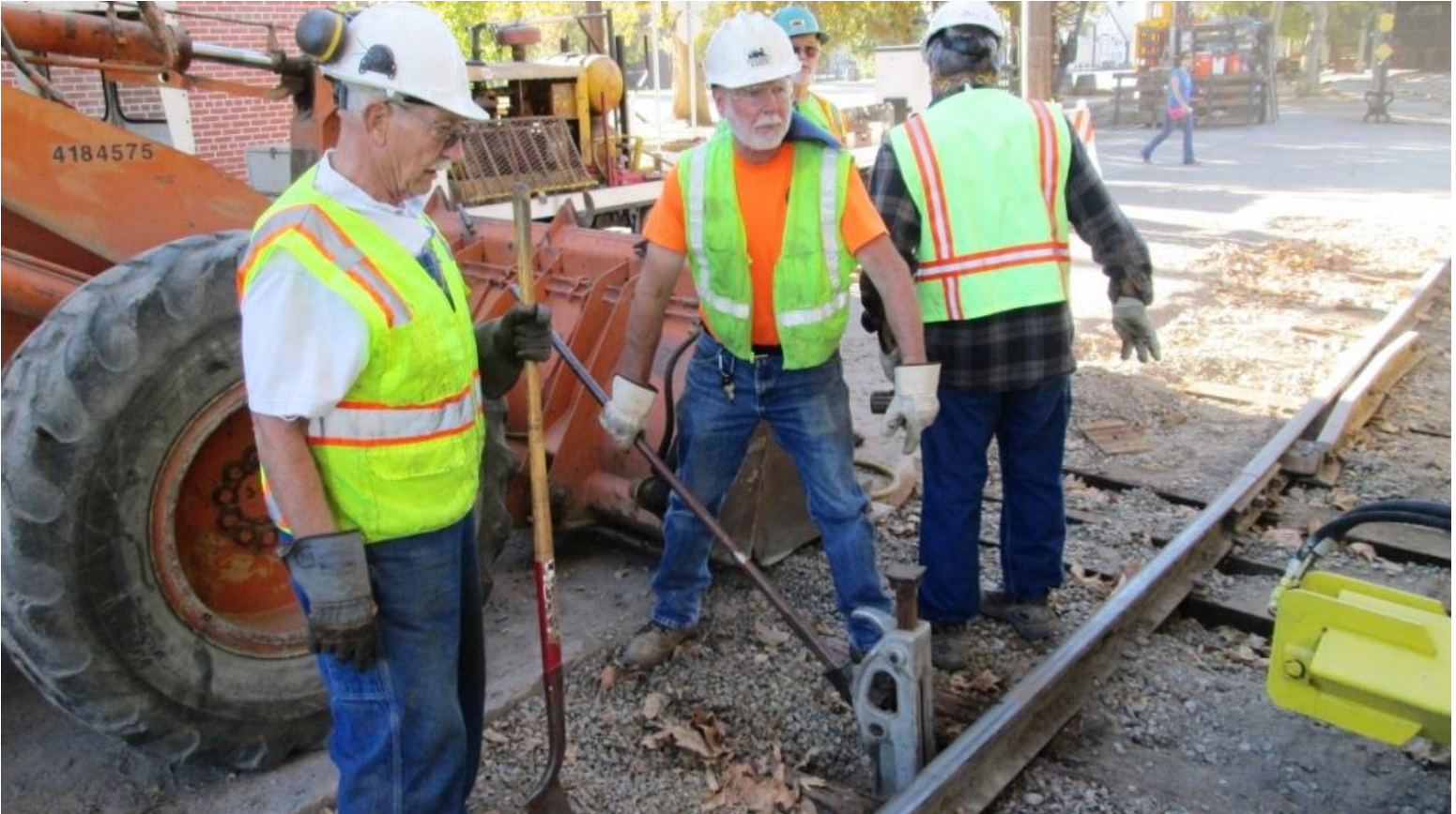
Mike M. and Clem jack-up the east rail just enough to relieve downward pressure on the tie to be removed
