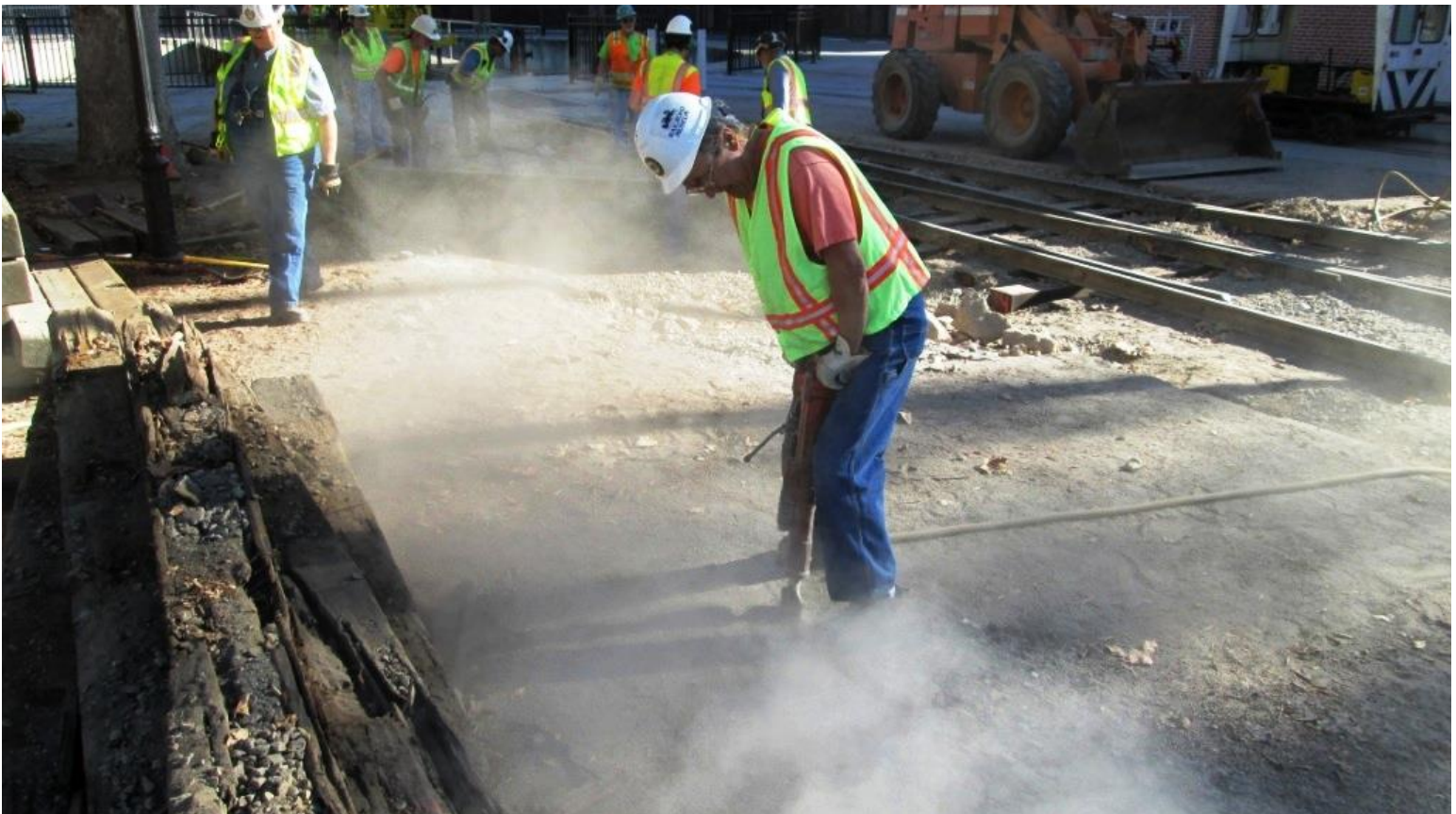
John kicks some dust up when breaking up the soil-cement with the jackhammer
